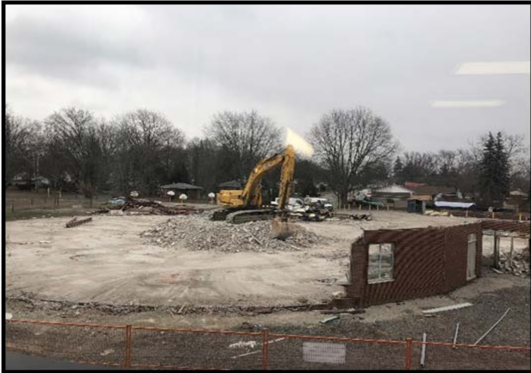
January 15, 2019 – Fairview Demolition
