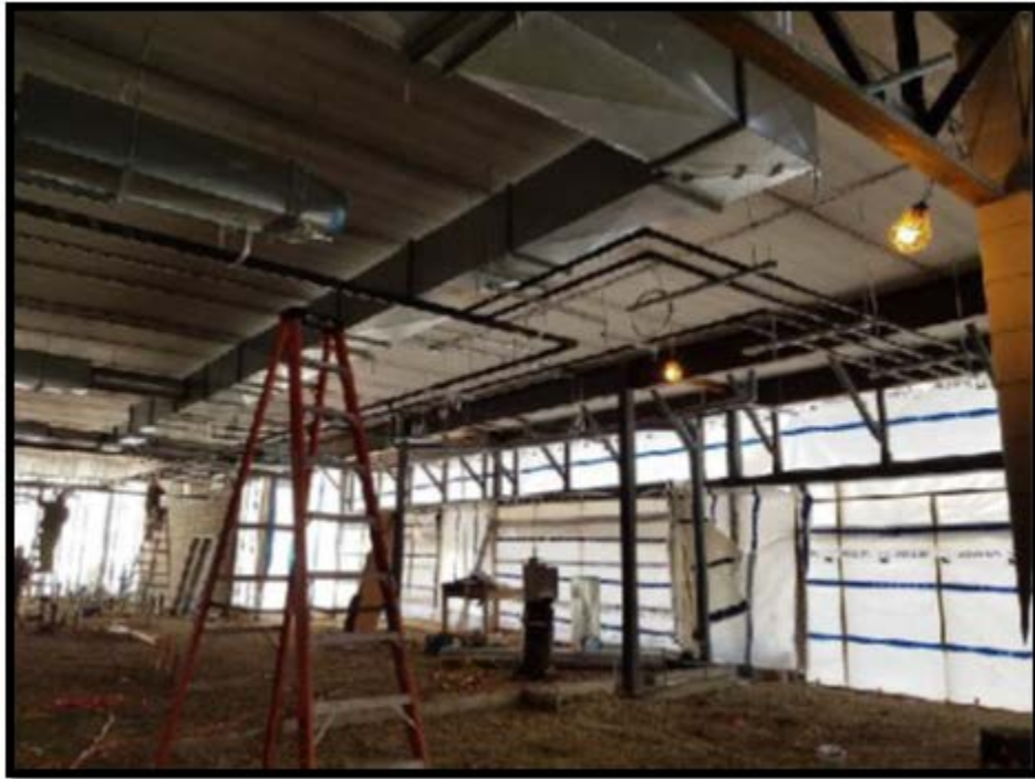
View of Kindergarten spaces. HVAC rough-in is nearing completion.
